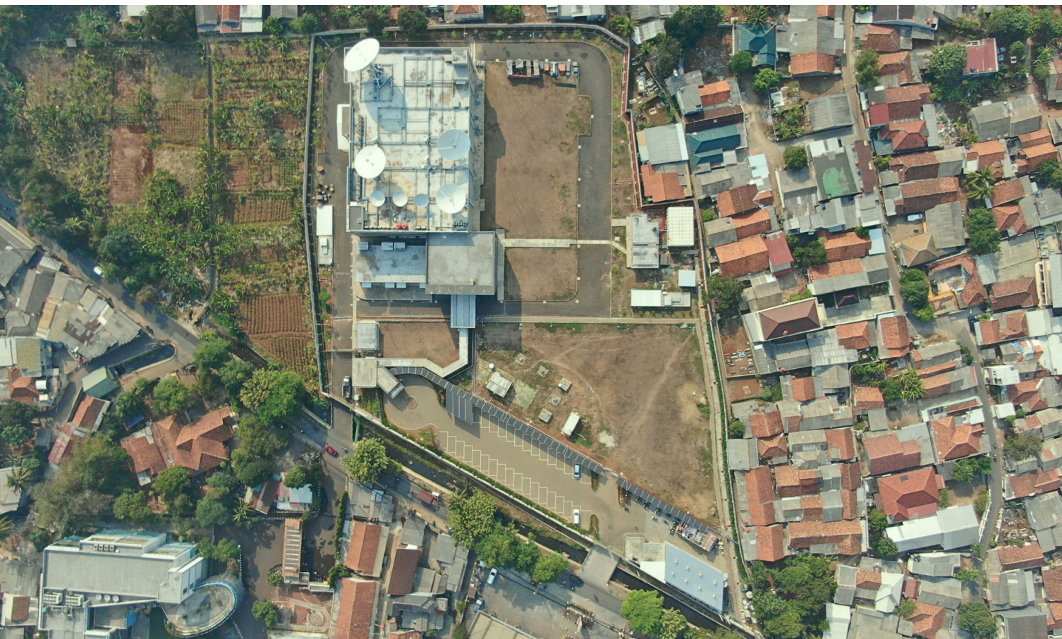
Tampak via udara AREA31 Cimanggis Aerial view of AREA31 Cimanggis
